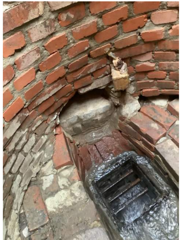
Figure 8 – CSO 110 Diversion Weir Photo
