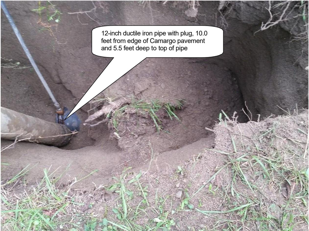
Several locations require SUE locating of existing underground utilities to refine the design for 60% as follows – the findings have been added for 60% BDM update. One pipe collapse on the stormwater system was found and reported to the City of Madeira.
