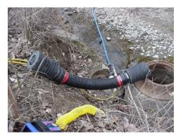
2. Fill the manhole to the top of casting and maintain this level for a period of at least 30 minutes. This is to allow exfiltration out of the manhole to fill the voids in the soil surrounding the manhole in dry periods in order to simulate a high groundwater condition.
