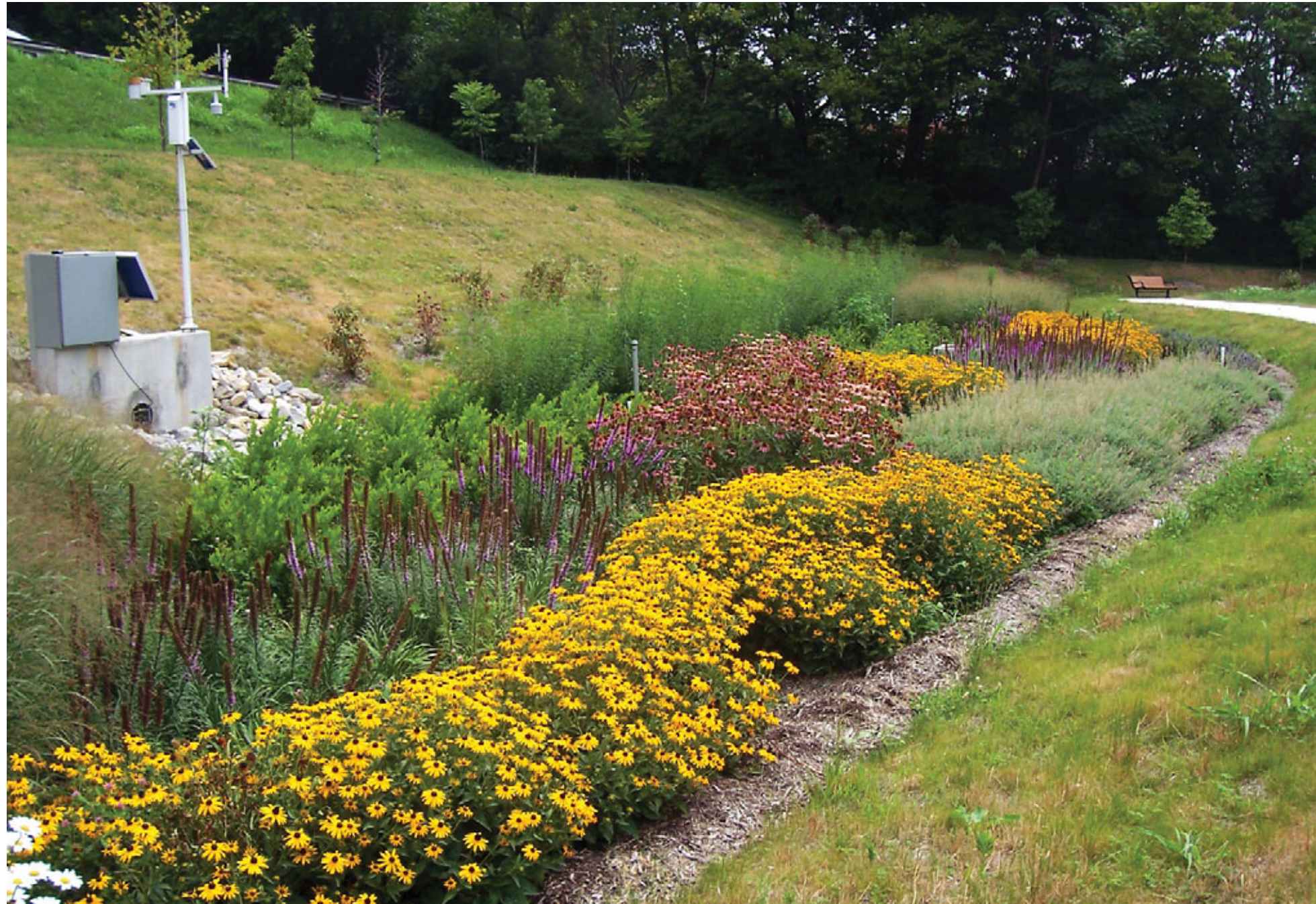
St. Francis Bioinfiltration Basin (2011)
