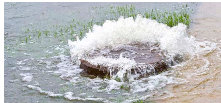
Excess flow in combined sewers can cause sewer backups in homes and businesses.
