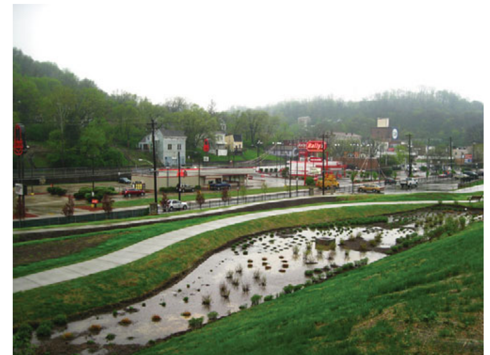
St. Francis Bioinfiltration Basin during a Rain Event
