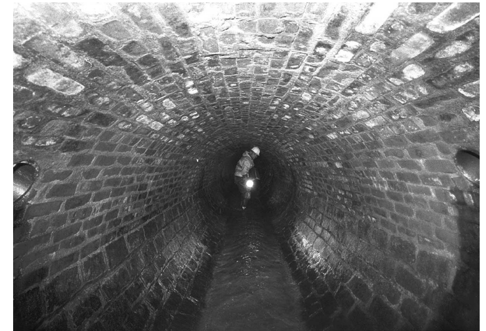
Brick sewer from the 1800s
