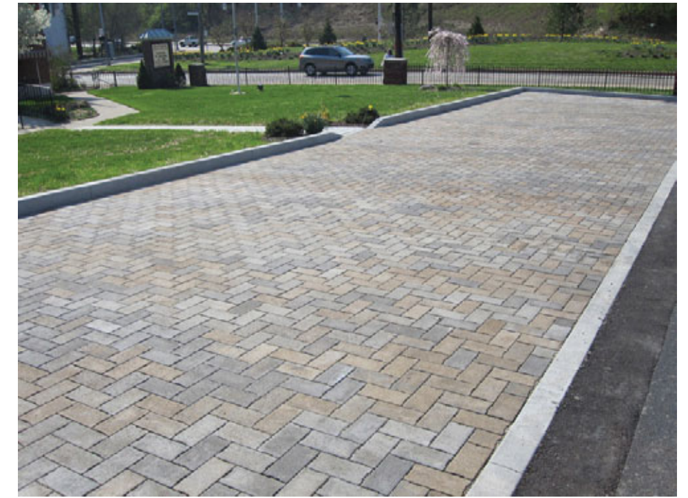
San Antonio Site After Installation of Permeable Pavers
