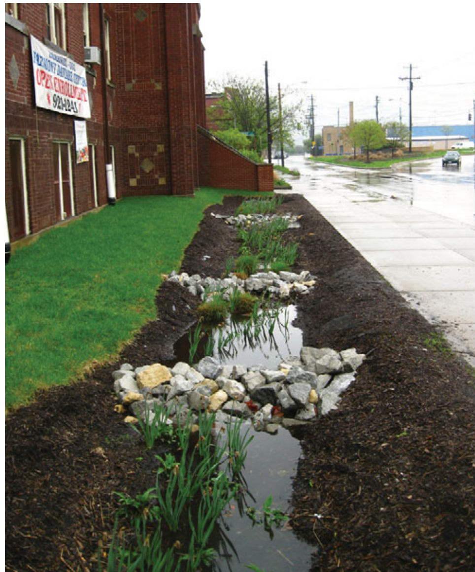
Bioinfiltration Basin at Immanuel United Church
