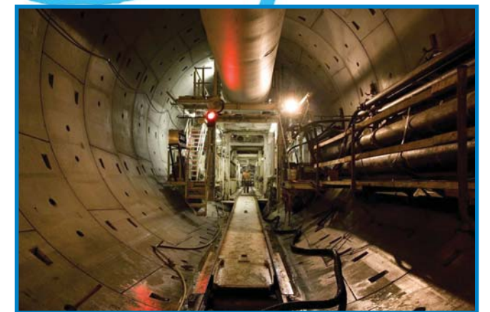
A look inside a tunnel.
