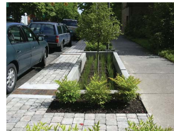
Integrated Stormwater BMPs
