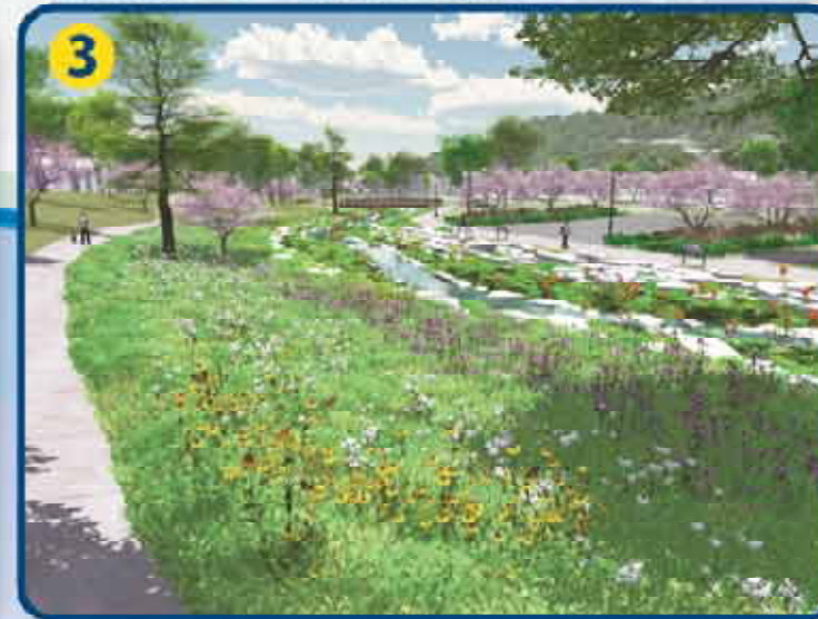
(Looking Northwest) This image depicts the character of the proposed urban waterway near the Civic Recreation Hub. Native vegetation is included to help reduce maintenance needs and to provide water quality benefits during high flow events. The pedestrian bridge in the background is above the modeled 100 year floodplains elevation; so during large volume rain events, water elevations would be contained within the heavily-planted areas.
